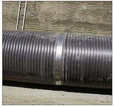
Weholite flexible couplings. The 40 foot lengths of 120" Weholite are the largest HDPE pipe joints installed anywhere in the world.
